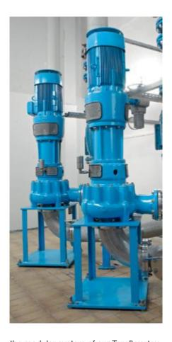
the modular system of our Turo® vortex pump. All types of design (submerged, dry mounted with vertical and horizontal configuration, close-coupled or bearing frame pumps, shaft or cantilever) are available.
