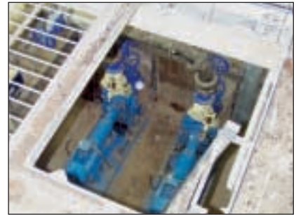
The compact design of the B pumps are making cellar applications possible.
