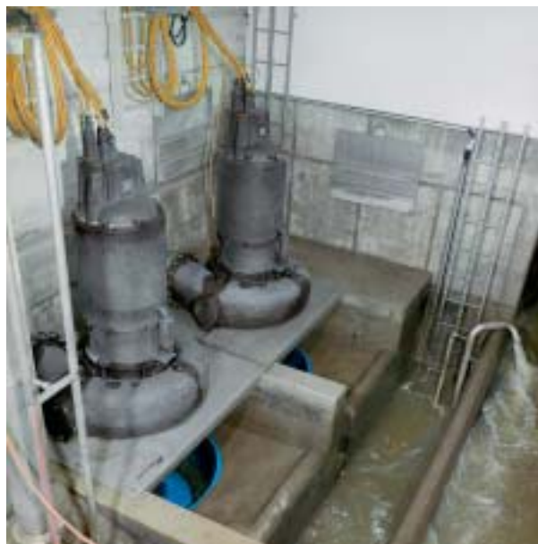
Rainwater pumps with the PREROSTAL® System.
