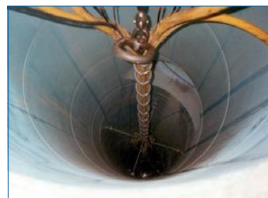
Fig. 3.3-b: Example of a rope with cable holder for an installation depth of 50 m
