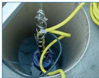
Fig. 3.3-e: Cable attachment using simple cable straps
