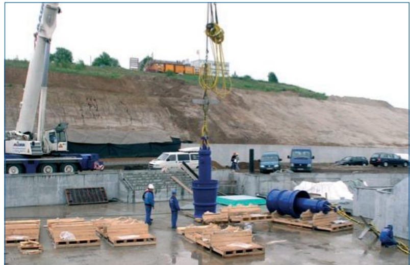
Fig. 1.1-i: Installation of submersible motor pump with a mobile crane
